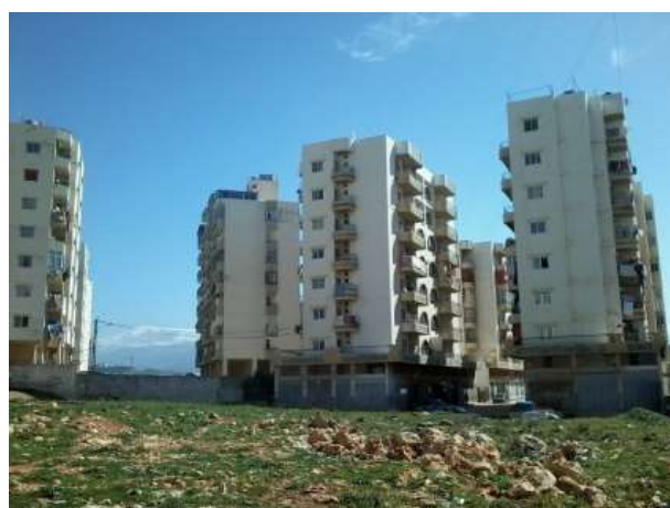
Figure 12: Typical apartment blocks in Kobbe
