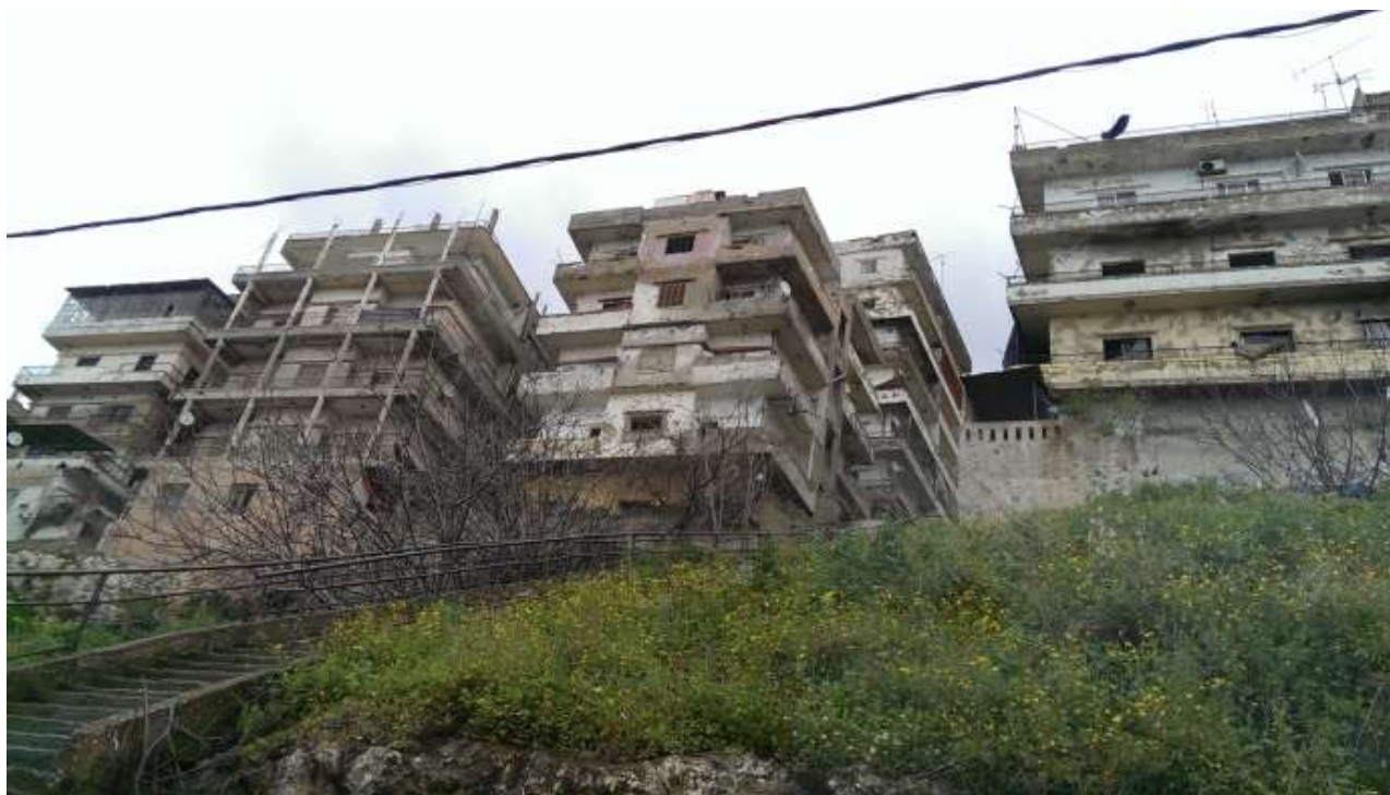
Figure 10: Housing in Jabal Mohsen showing damage from bullets
