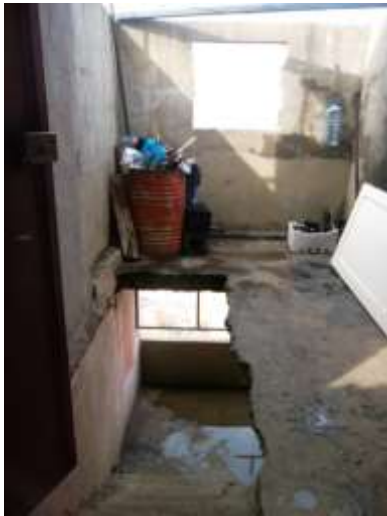
Figure 25: Stairwell in Mankubin
