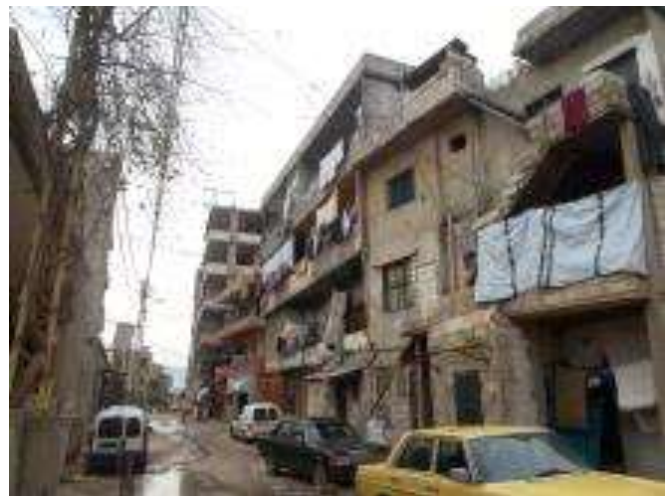
Figure 14: Poorly constructed apartment building in Shalfeh
