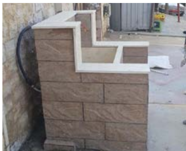
Figure 7: New water point in Baddaoui completed. ©Akkarouna
