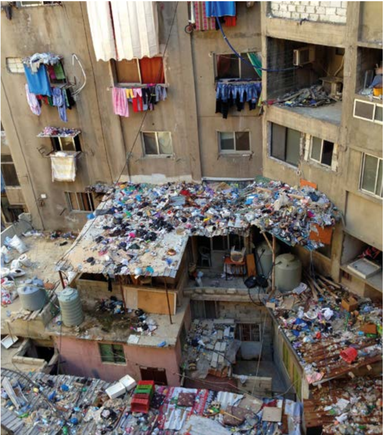
Figure 14: Photograph showing waste disposal in the immediate vicinity of the housing block in Tabbeneh ©Adel Sarkozi/CARE
