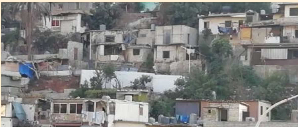
Figure 17: View of new street lighting and walkway rails in Malawieh ©Hussein Zeidan CARE 2019.
