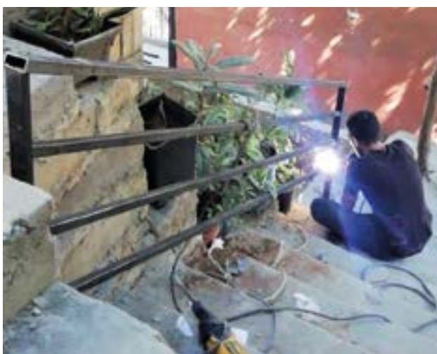
Figure 6: New staircase Malawieh. ©Akkarouna
