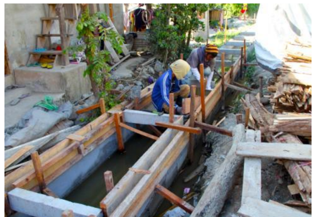
Photo 3: CFW workers drainage canal in Barangay Kauswagan, Cagayan de Oro City Source: Afrhill Rancel, IFRC
