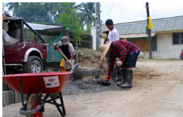
Photo 2: Cfw workers drainage canal in Barangay Upper Hinaplanon, Iligan City Source: Afrhill Rancel, IFRC
